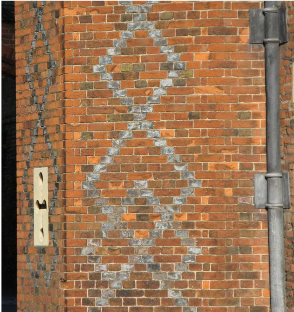
Diaper Brickwork Burnt Headers formed in a diamond pattern
