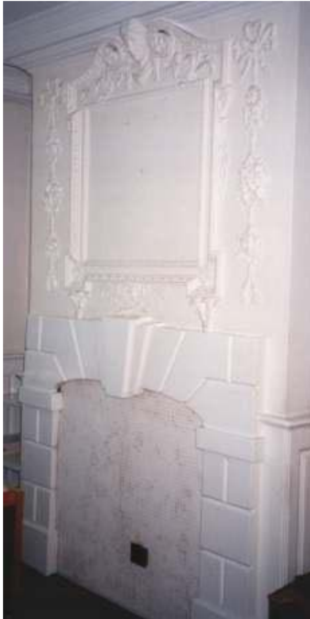
This unusual rusticated fireplace of the early 18 th century has an overmantel above in a hogarthian baroque style.
